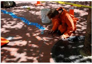
Fixing the weathered expansion joints in the sidewalk.
